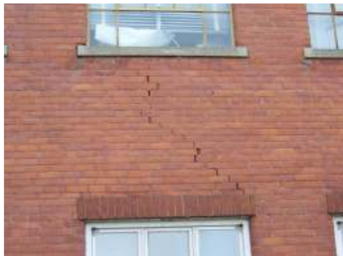
Photo 2 – Stepped Cracks in Brick (West Elevation)
