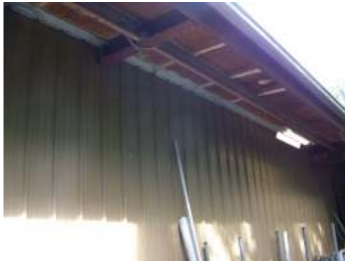
Photo 9 – Exposed Framing at PEMB Eave (North Elevation)
