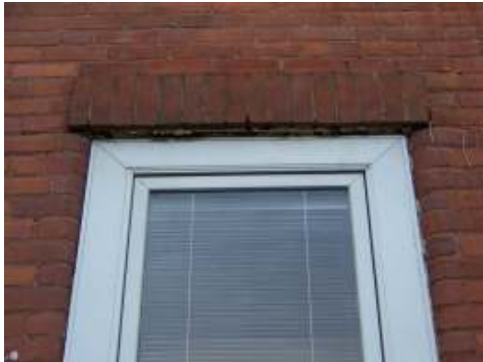
Photo 3 – Deteriorating Steel Lintels (West Elevation)
