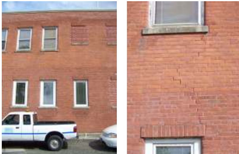
Photos 5 & 6 - Stepped Cracks in Brick (East Elevation)
