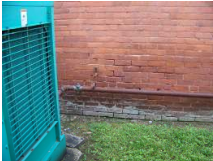
Photo 4 – Brickwork Requiring Repointing (West Elevation)
