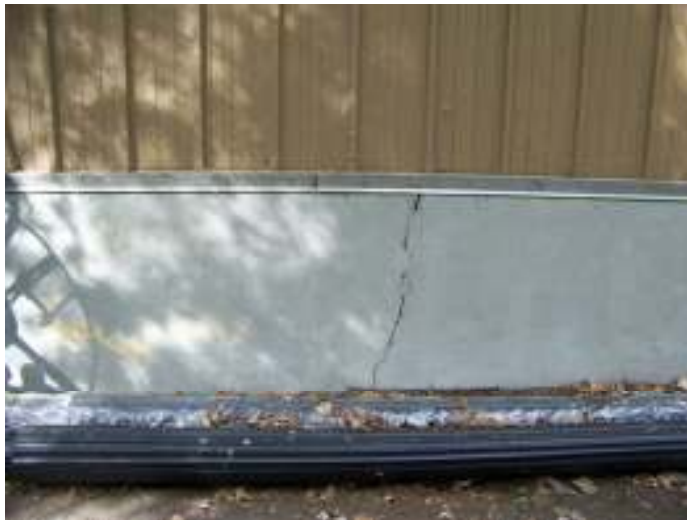
Photo 10 – Crack in Foundation Wall (North Elevation)
