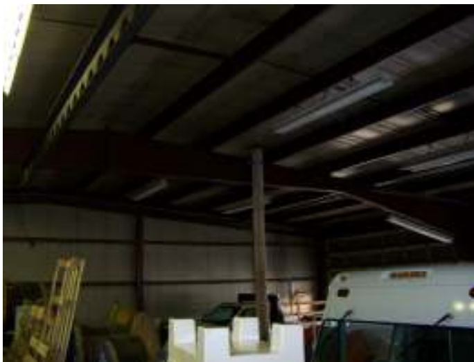
Photo 18 – Close Ups of Tapered PEMB Frames and Purlins (Main Garage)
