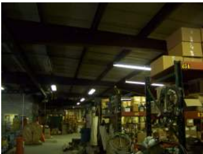
Photo 14 – Tapered PEMB Frames at Elevated Dock (Main Garage)
