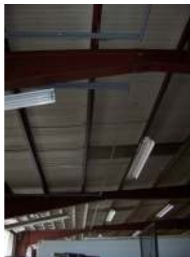
Photos 16 & 17 – Close Ups of Tapered PEMB Frames and Purlins (Main Garage)
