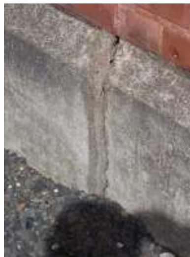
Photo 7 – Foundation Crack (East Elevation)
