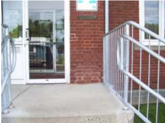
Photo 8 - Brickwork Requiring Repointing/Repair (South Elevation)
