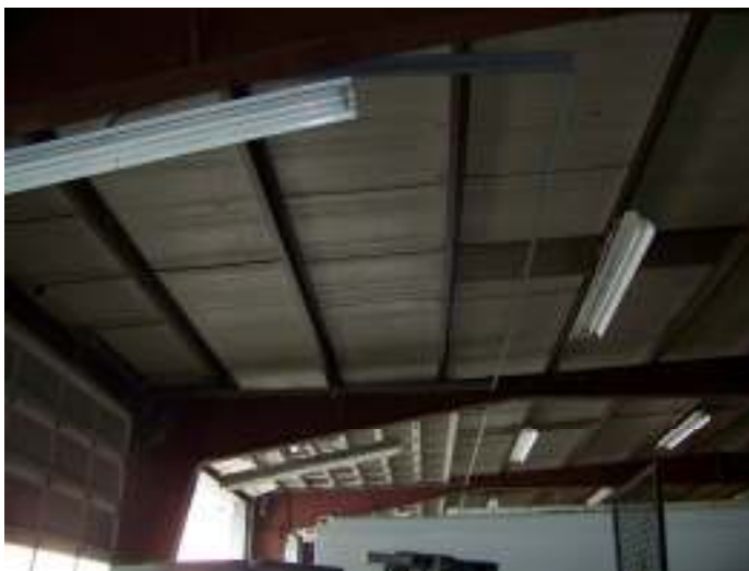
Photo 15 – Tapered PEMB Frames and Purlins (Main Garage)
